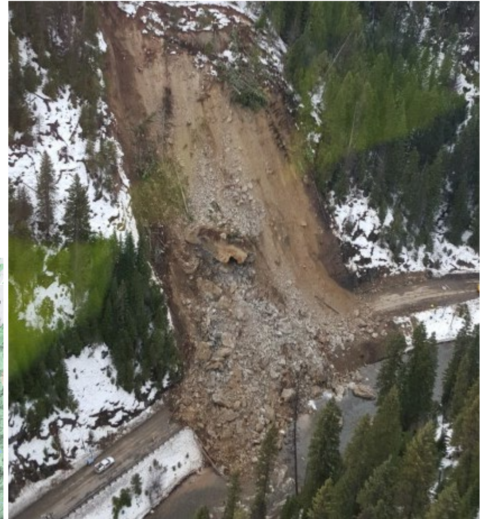
2016 Elk City Landslide on state highway (video link)
